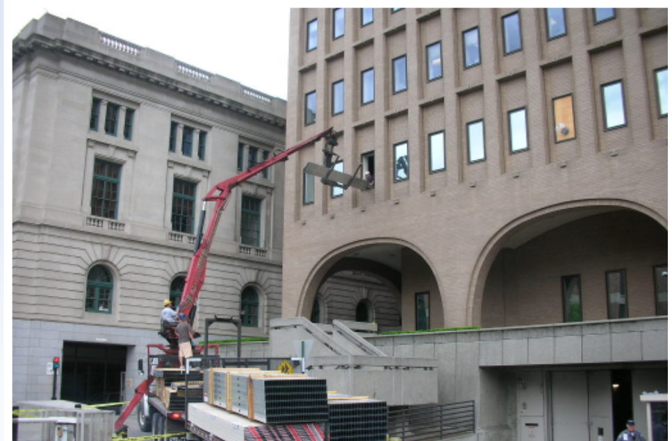
Working in an occupied building presented challenges
